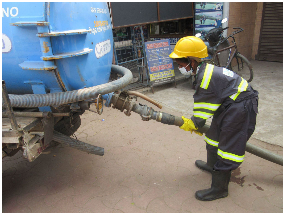
Figure 6: Women engaged in septic tank cleaning with access to adequate support through the professionalisation of the occupation under the Garima Scheme in Odisha, India (Photo: Jhunulata Naik)
